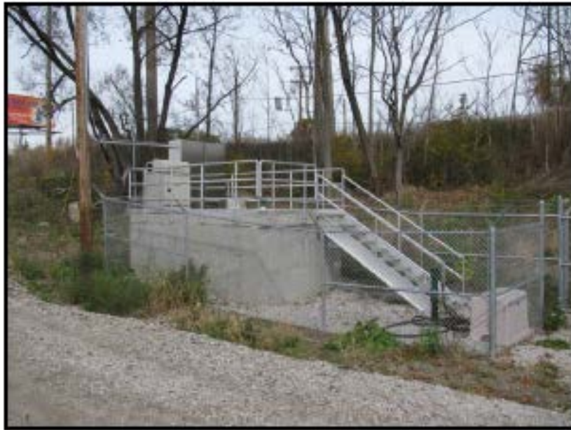
Figure 4, CSO Station 003 Photo
